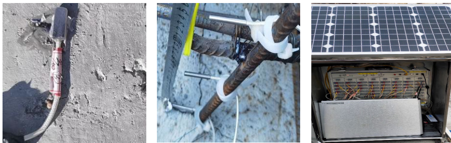
(a) Thermometers on the top edge of the ballastless track
